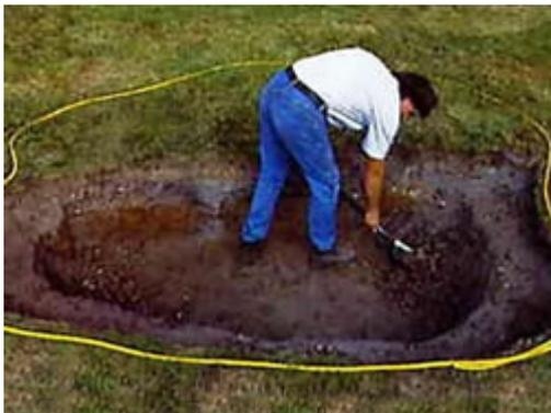
Excavate the pond evenly down to the depth of the marginal shelves. These must be deep enough to accommodate a marginal planting basket. Then excavate the full depth of the pond, digging down from the marginal shelves to create the deepest area of the pond.
