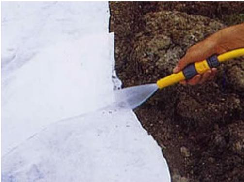
Dampen the underlay so that it clings accurately to the shape of the excavation. This makes it easier to install the pond liner. The underlay is then smoothly contoured and there is little chance of it causing wrinkles beneath the liner.
