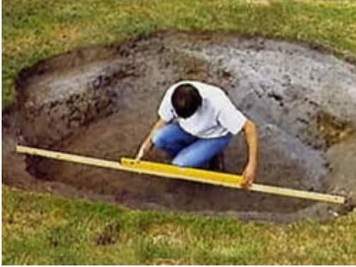
It is vital that the marginal shelves as well as the edge of the pond is level from side to side and end to end. If the pond is not level, then the liner will become exposed in the higher areas, while there is a likelihood of water spilling over the lower edges and flooding the surrounding ground.
