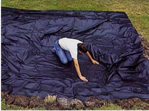
Smooth the liner to the contours of the excavation, working from the floor in the centre outwards, removing as many creases as possible. Where there are awkward angles or corners, make a single bold fold, rather than several smaller ones.
