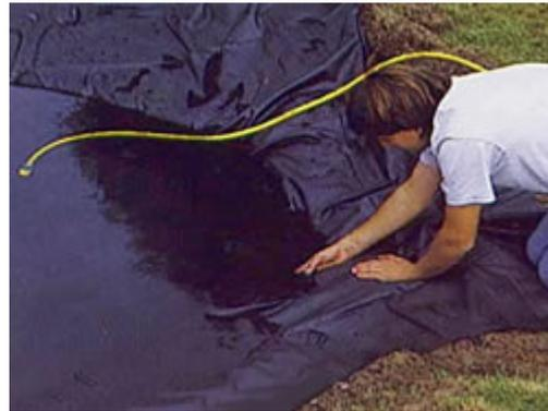
Once the pond has been filled, the edge of the liner should be trimmed and an edging provided.
