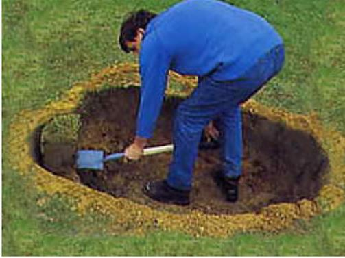
Dig out the excavation making it as accurate as possible. Ensure that when calculating the depth, an additional 3 to 5cm is allowed for a cushion of sand on the shelves and floor to support the pond.
