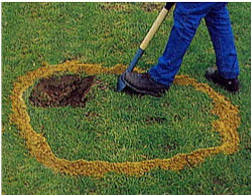
Remove the pond and commence digging. Dig down to the depth of the marginal shelf across the entire excavation. Add approximately 5cm all around the excavation to allow for the tapering shape and back-filling.
