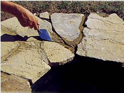
Make a mortar mix of four parts by volume of bricklayer's sand and one-part cement with water mixed in until it is a sticky agglomeration. Lay paving on a bed of mortar so that the paving is level and provides a small overhang. Then point with mortar between the stones.
