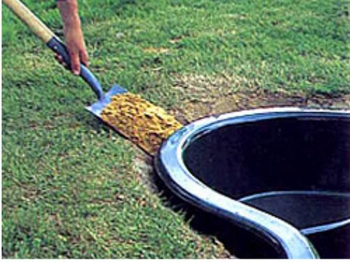
Back-fill with sand to provide a cushion all around. This is preferable to using excavated soil as it will flow evenly and provide proper support. The back-filling must be done evenly around to ensure that the pond does not move or twist in the process.
