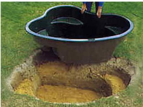
Carefully lower the pond into the excavation. Make any adjustments that are necessary to ensure that it sits squarely. Make sure that there is sufficient space all round for back-filling with sand.
